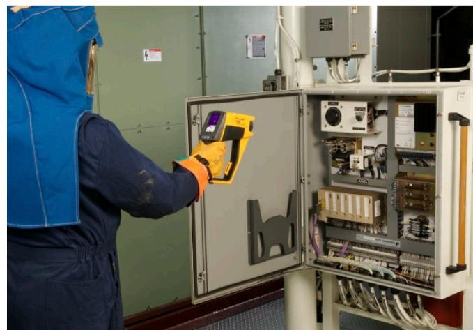
The thermal imager also helped to track down some overheating problems. The first had to do with the voltage regulators for the big generators that provide the electricity that runs the ship. "The voltage regulator for that system kept
